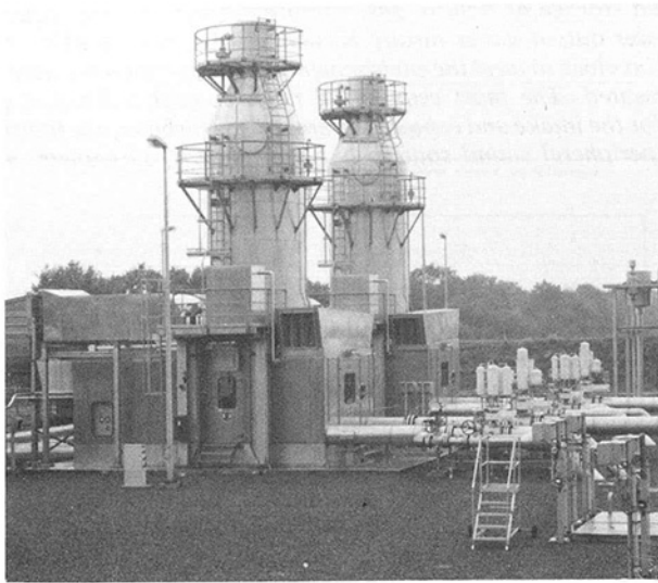
Fig. 3 Engine house in lightweight construction
