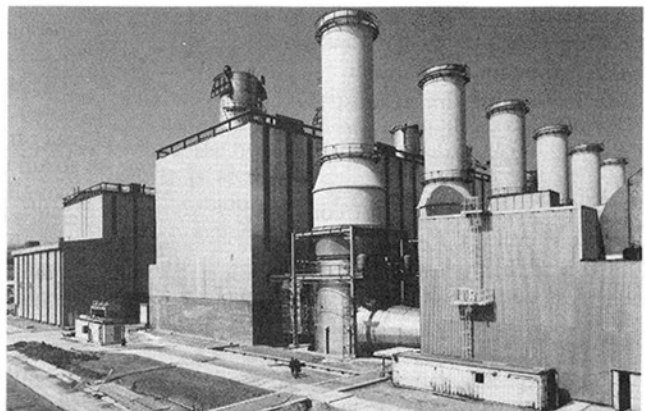
Fig. 1 The 1350-MW Ambarli GUD power plant under construction
